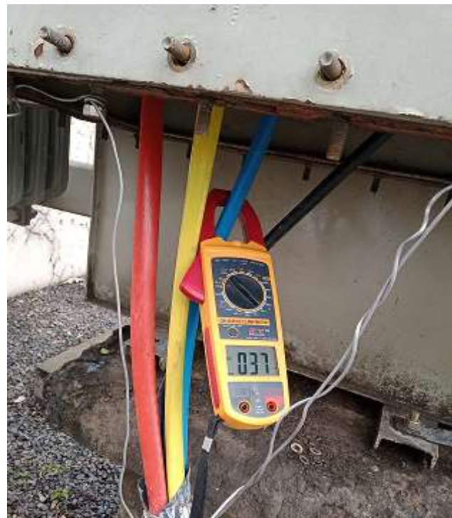
Fig. 5.2 Admin block power measurement
